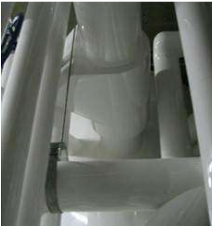
Cold insulation for Cryogenic System - LNG or Gas processing
