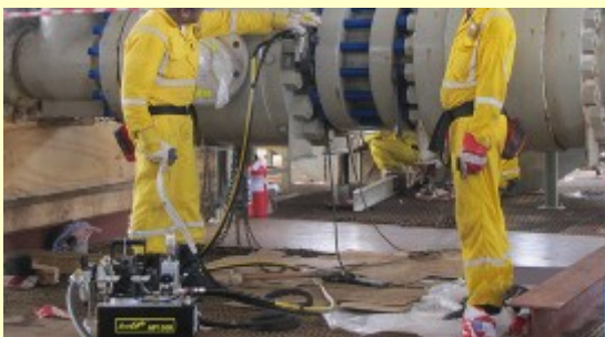
Figure 4 : Flange Hydraulic Torque Wrench (HTW) in use
