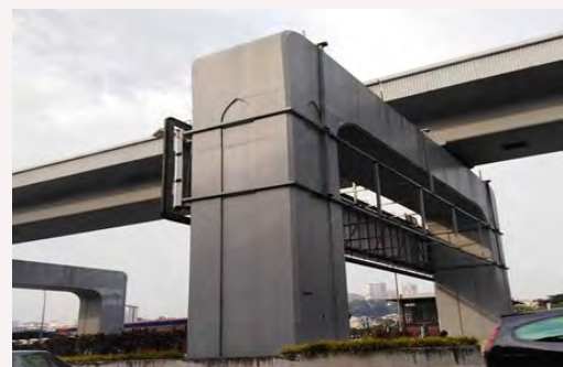
Figure 23 Anti Carbonation Paint on the Piers of MRT in Bangsar
