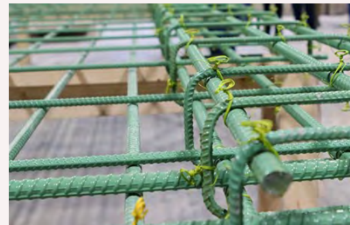
Figure 28 Epoxy coated rebars
