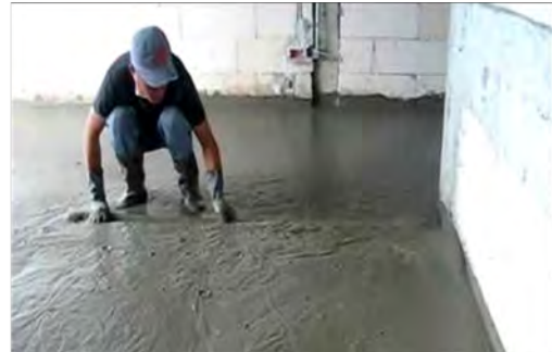
Figure 18 Adding mortar or concrete
