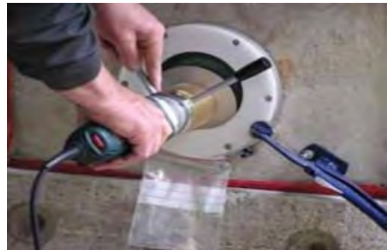
Figure 15 Extraction of Samples for Chloride Testing
