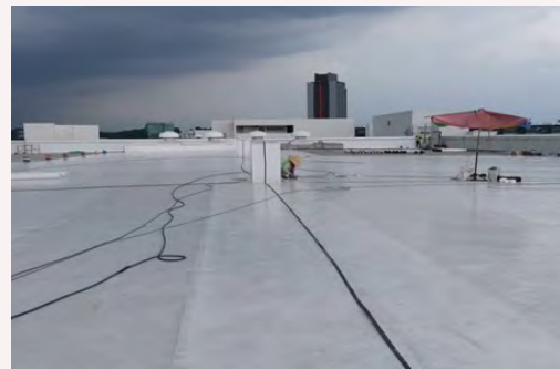
Figure 22 Single ply membranes against water ingress
