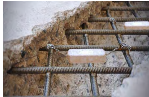
Figure 27 Zinc based sacrificial anodes
