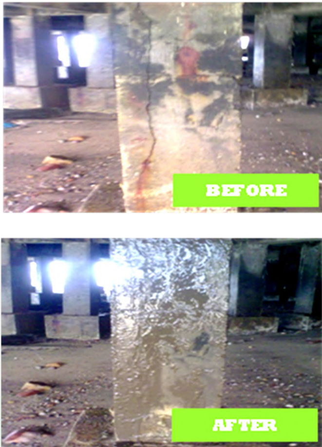
Figure 2 Application geopolymer coating on site; (a) Before coating, (b) After coating
