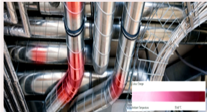
Figure 4: Thermal Indicating Coating with an irreversible colour change at 60 to 80 °C to red (Visual inspection to identify wet insulation/damaged insulation) without the need to open the cladding.
