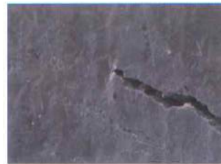
Fig 5: Stainless Steel heat exchanger plate showing blunting at the crack tip
