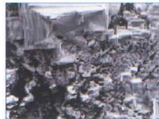
Fig 6: Corroded surface of a low alloy steel pipe
