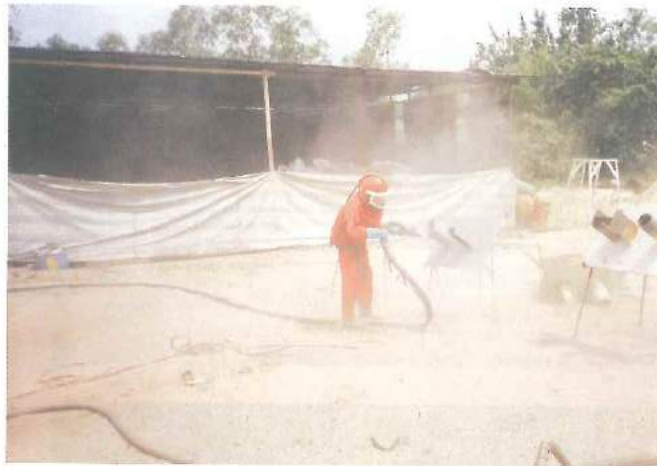
PRACTICAL TRAINING/ASSESSMENT IN PROGRESS (BLASTING OPERATING)
