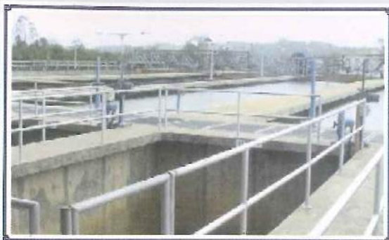
A side view of the Plant - Treatment Area
