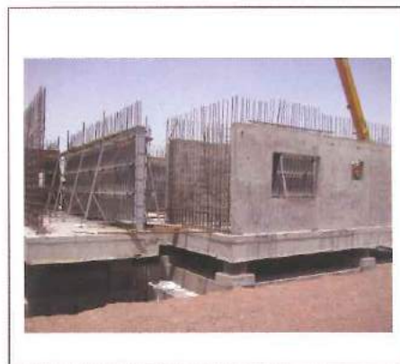
Construction of the first floor after the bearing installation
